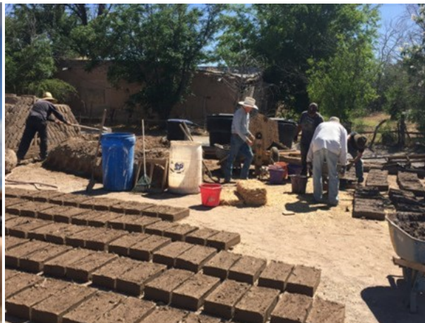
Fig. 15 Making adobes in Mesilla, New Mexico, USA
