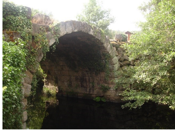
Fig. 79 Arquinho bridge, in Valpaços (source: photo of the author).
