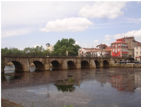
Fig. 81 Trajano Bridge, in Chaves (source: photo of the author).
