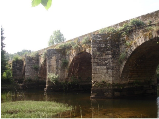
Fig. 78 Stone bridge, in Mirandela (source: photo of the author).
